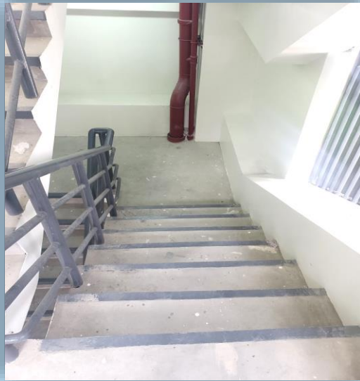
Hallway, Lift Lobby and Fire Exit
