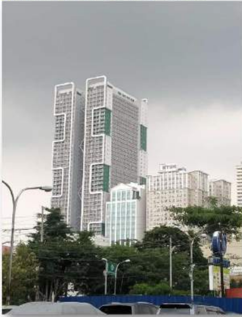
BUILDING FAÇADE : ALONG AGNOS ST.
