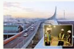
NLEX Harbor Link Segment 10
