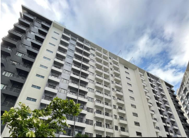
TOWER 2 FACING AMENITY
