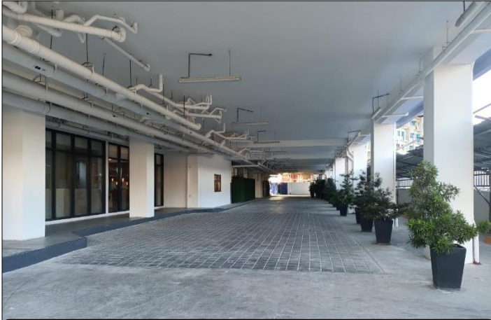
DRIVEWAY AREA AT TOWER 3
