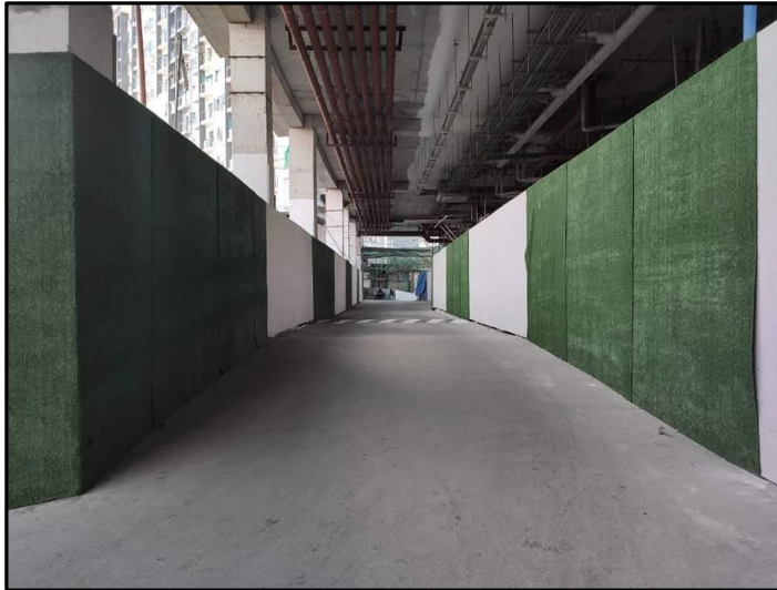
DRIVEWAY AREA AT TOWER 4
